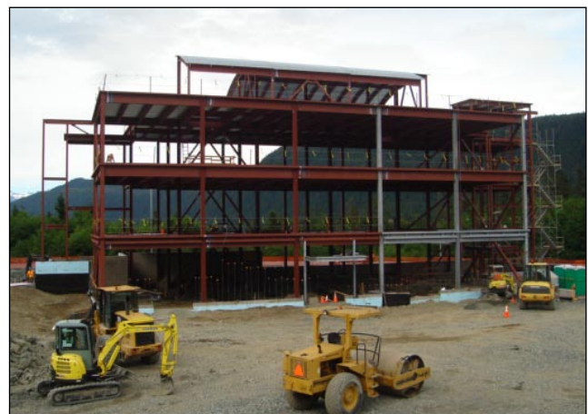
The Lena Point Fisheries Facility in late July 2007. Photo: Karl Petterson.
