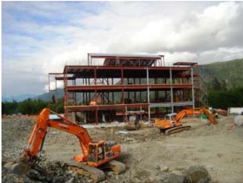
Lena Point construction, Aug 22, 2007, by Karl Petterson
